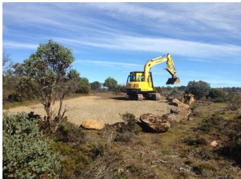
Construction of a vehicle barrier at Skullbone Plains
