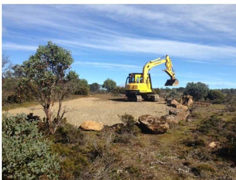
Construction of a vehicle barrier at Skullbone Plains
