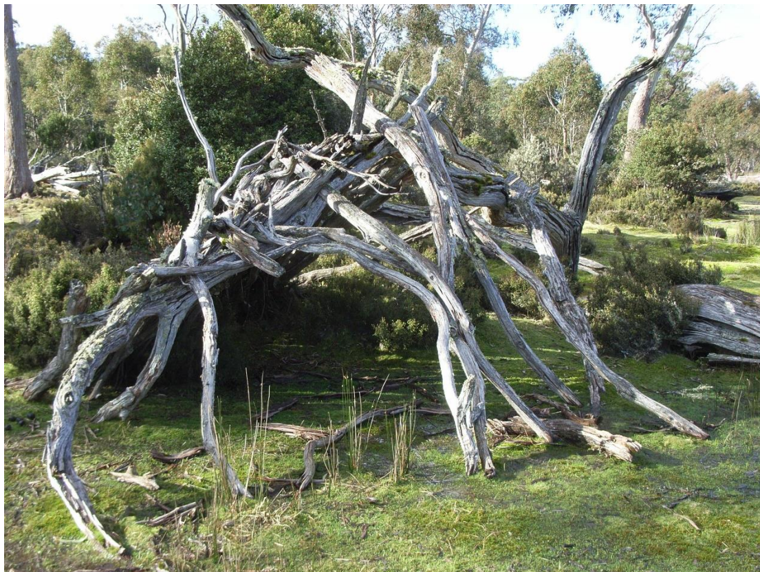
Figure 3 Aboriginal mia-mia found by John Wilson and Peter Sims in the northeast corner of the grassy wetlands in 2009. It is likely that this structure was close to two hundred years old.
