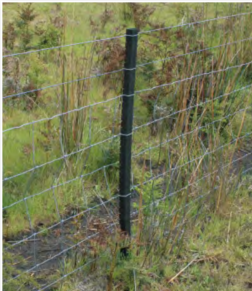
Poly dropper used to tension between widely spaced posts, King Island (Garry Sutton)
