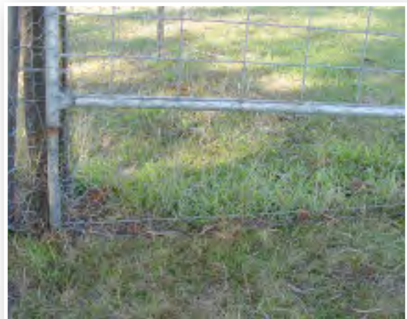
Wire and mesh added at bottom of gate on sloping land, Gunns Plains (Colin Vercoe)
