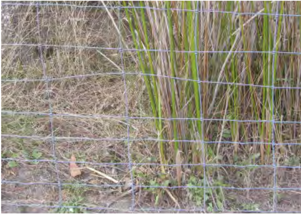
Mesh with knot B showing wires forced apart by wallabies (Geoff Dean)
