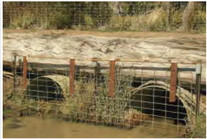
Free-swinging gates on culvert, Forestier Peninsula (Matt Dunbabin)
