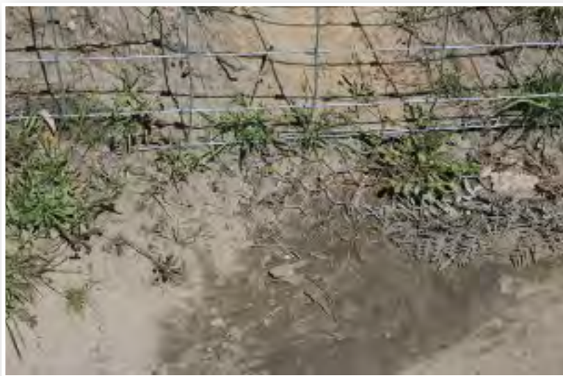
Rabbit netting attached to bottom of wallaby proof fence, Mt Lloyd (Joe Blair)
