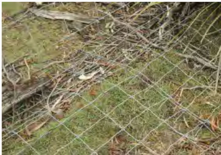
Fence mended to replace rusted bottom wire, Pipers River (Brian Baxter)
