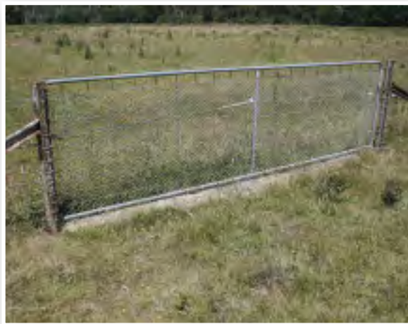
Concreted gate sill, Waverley Farm, Mathinna
