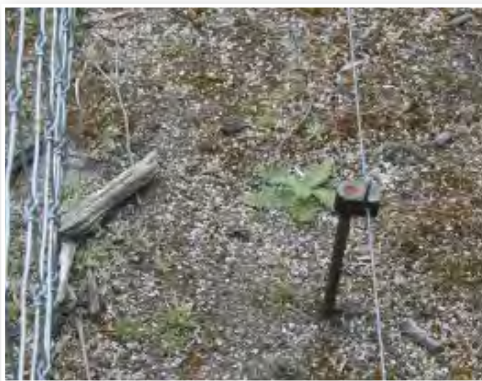
Low offset electrified outrigger, Goulds Country (Shirley and Norm Rattray)
