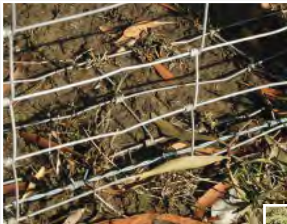
Fence bottom wires bent flat, Tasman Peninsula (Guy Dobner)
