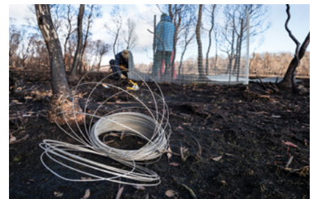
Installing fences at Five Rivers. Photo: Heath Holden
